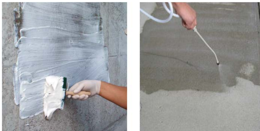
Figure 2-30: Silane based cream (left) and liquid (right) (Sika, 2016)
