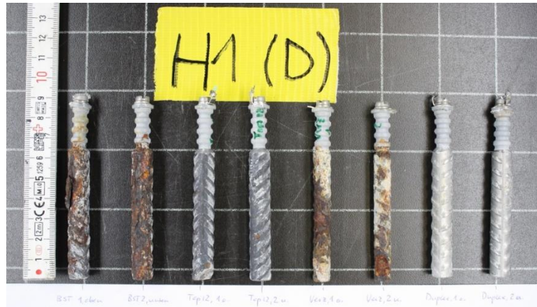
Fig. 8. State of corrosion of the rebars in concrete after 12 years chloride exposure and carbonation for plate H1 with cover thickness of 10 mm. From left to right: 2 x carbon steel B500B; 2 x TOP12; 2 x galvanized B500B; 2 x stainless steel 1.4462.
