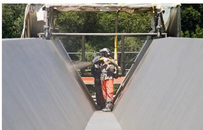
Membrana bicomponente Sikalastic®-851 R<sup>1)</sup>
