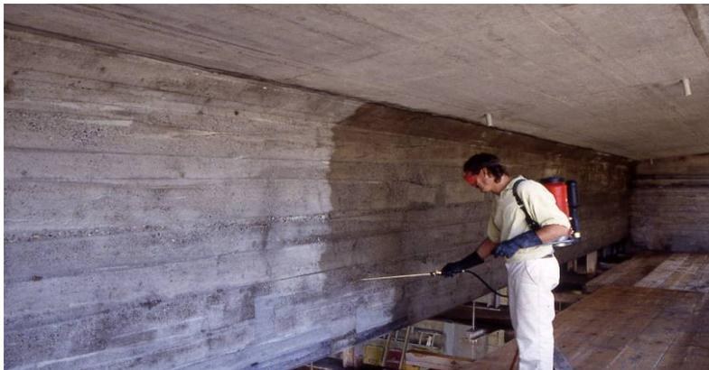
Fig. 7 Application of Sika FerroGard-903 by low-pressure spray
