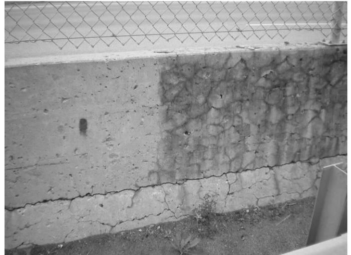
Figure 2. Silane-treated (left) and untreated control (right) median barrier segments near Québec City, Canada.
